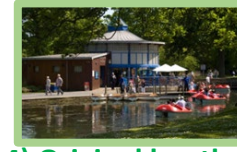
4) Original boathouse removed and rebuilt
