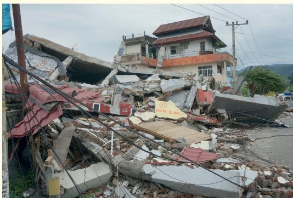
The photograph above shows the damage caused by an earthquake in Indonesia a Low Income Country.
